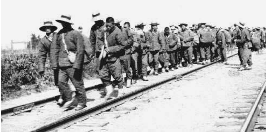
Figure 14. Chinese workgang on CPR track.
