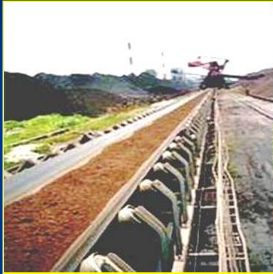
Conveyor belt feeding a stacker/reclaimer
